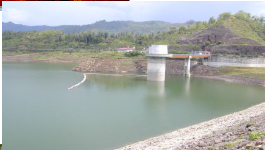
Serma dam, Yogyakarta, Indonesia View of the artificial lake. (Photo credit: E. Garcia-Agudo/IAEA)
